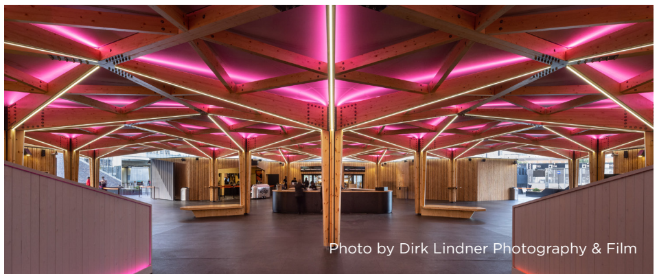
Structure showcasing the extensive use of Glulam and CLT
