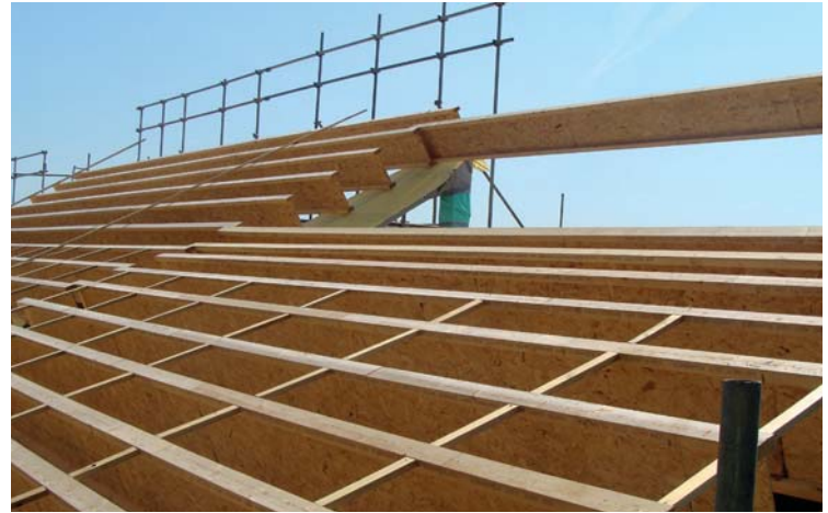
Construction of east wing
