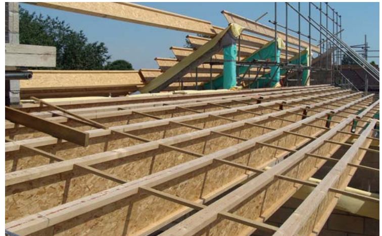
JJI-Joist roof being fixed to glulam structure
