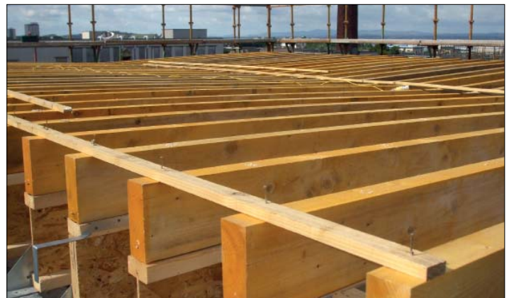
JJI-Joists used to create the gull shaped roof
