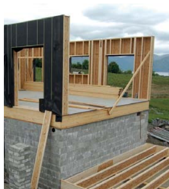
Lower floor commences with 400C JJIs
