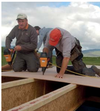
Maple Joiners fixing ply to 400C JJI purlins
