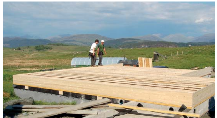
Constructing the main 400C JJI-Joist floor over the undercroft
