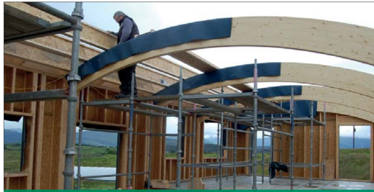
400C JJI purlins start on north side, over curved Glulam beams
