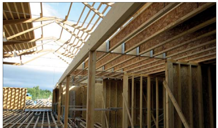
Ground, first and roof joists
