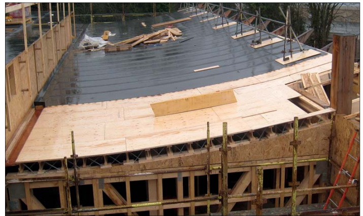
JJI-Joists used to create curved roof
