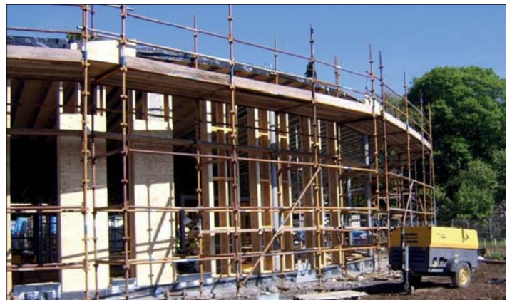
On-site construction of JJI-Joist wall panels
