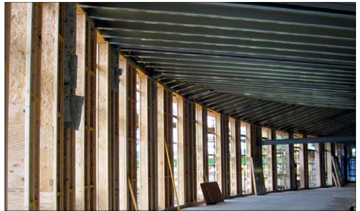
JJI-Joists forming the curved walls
