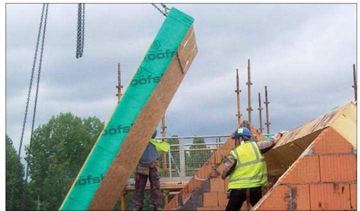
Roof cassette being lowered into place
