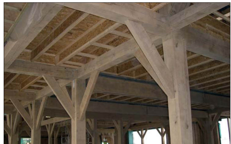
JJJ-Joists supported by oak frames
